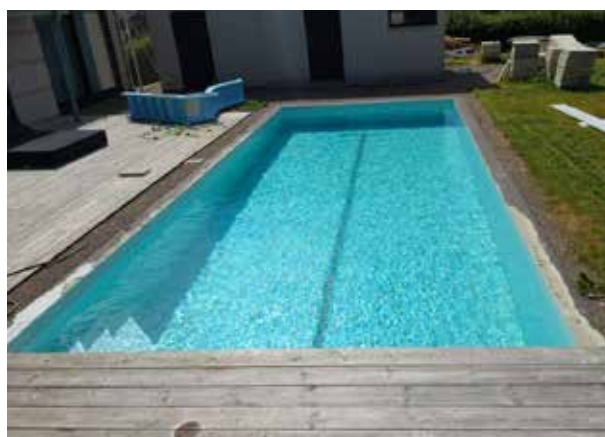
Privat pool utomhus i Viken: gjuten betong. System Sopro TDS 823.
